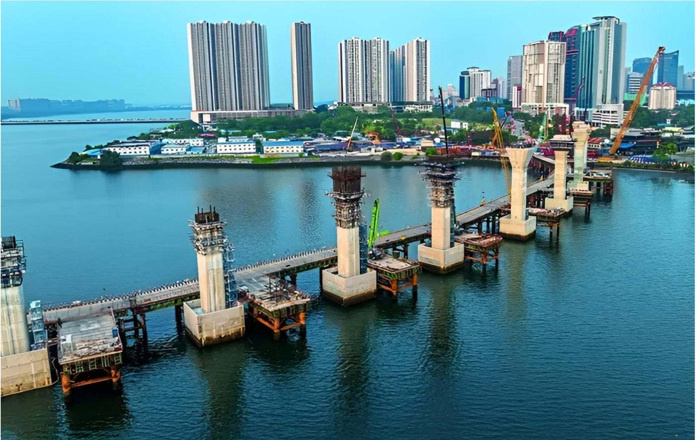
A railway viaduct is taking shape across the Strait of Johor. A trestle bridge has also been erected.
